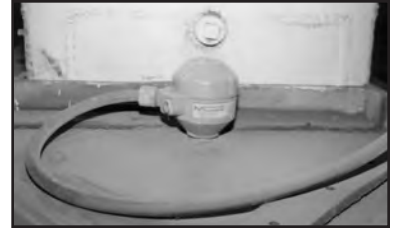
An installed SFD-2 in a coal-fired power plant provides an alarm output when there is an interruption in coal supply.
