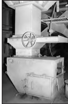
An installed SFD-2 in a coal-fired power plant provides an alarm output when there is an interruption in coal supply.
